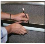
Position the profile, check the fit and mark the drill holes.
