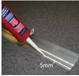
Apply 5mm bead to the underside of the profile, 2 lines for Single and 3 for double channel.
